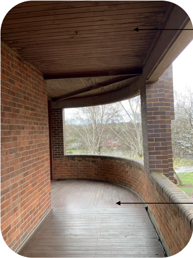
Salvage timber ceiling for re-use
